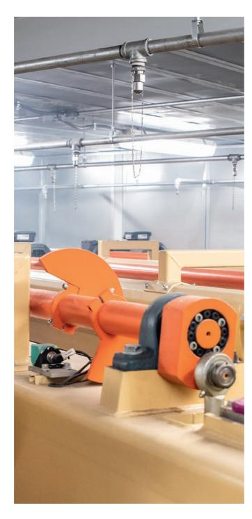
WoodTechProtect combines fire detection, water mist and spark extinguishing technology into a single system. Fire protection for wood processing machines is provided by Minifog ProCon water mist systems, while exhaust devices are best protected by spark extinguishing systems. Joint water supply and joint fire detection and extinguishing control panel can be provided for both systems.
