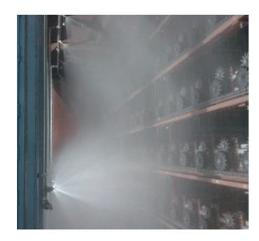
water droplets in the vicinity of the flame, which hinder the supply of oxygen to the fire. The extinguishing principle, which works by means of cooling- and smothering effect, allows particularly effective fire-fighting with reduced use of extinguishing water which also brings rapidly spreading fires under control.
